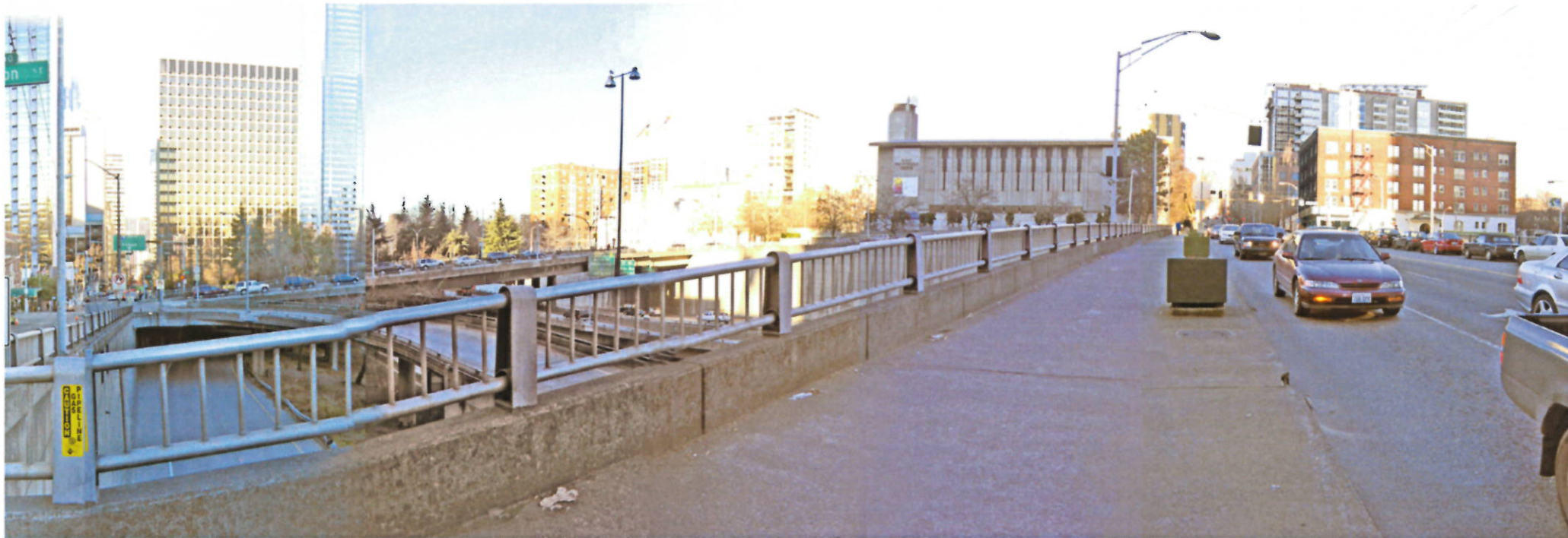
Figure A-2 Madison Street Bridge
